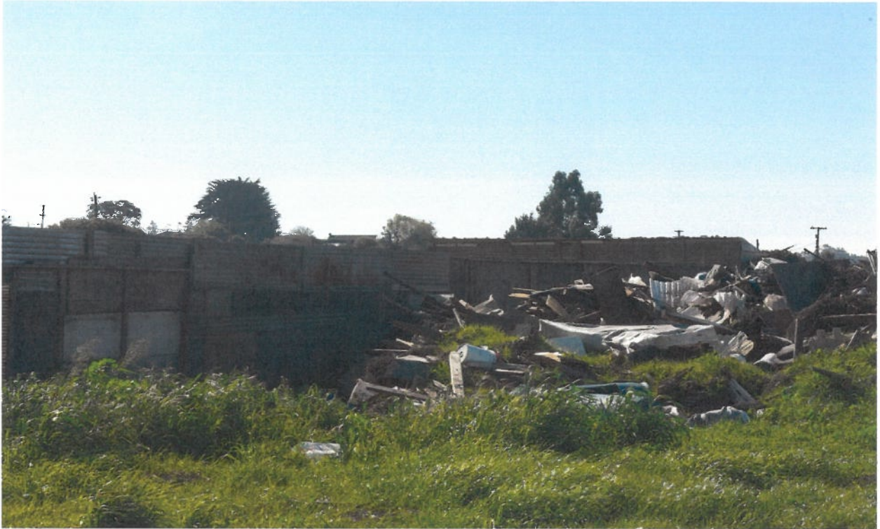
Debris pile after a portion of enclosures were demolished
