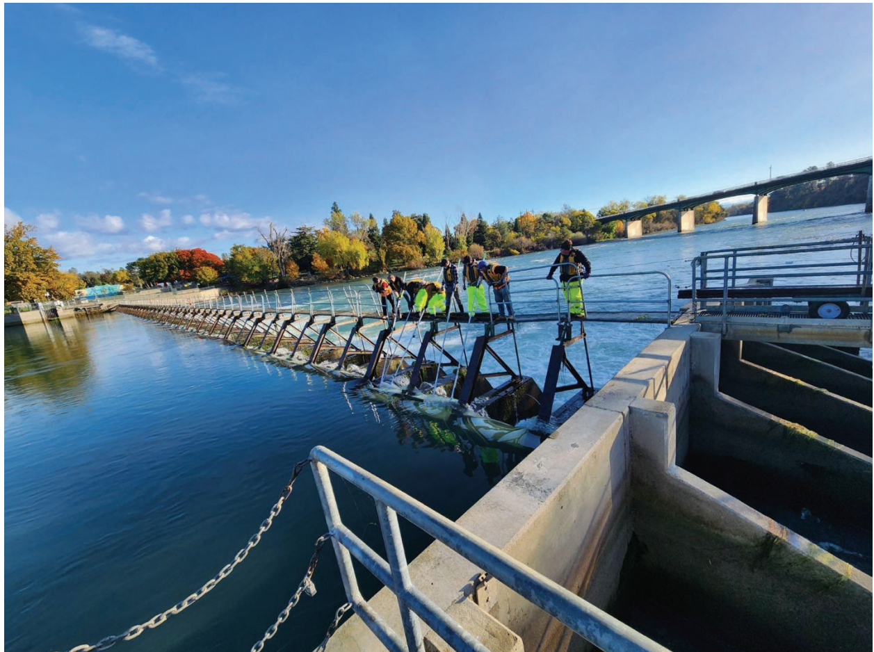
ACID employees erecting the diversion dam for another irrigation season. Photo used with permission by ACID Board of Directors.
